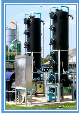
Manufacturing Plant Set Up
